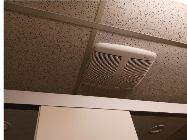
**Photo #M6:** Ceiling mounted ventilation fan.
