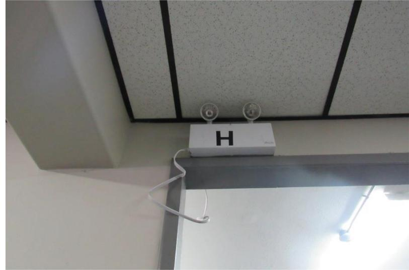
**Photo #E6:** Typical emergency battery pack.
