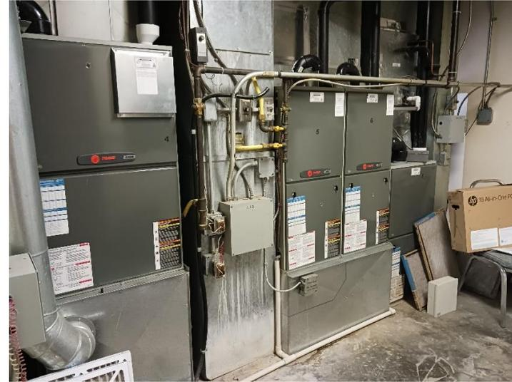
**Photo #M4:** Gas-fired furnaces in the bowling Alley.
